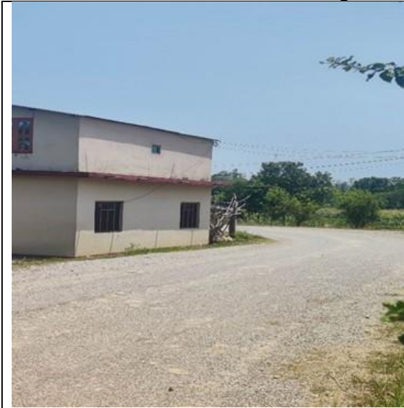
Figure 1: Affected load bearing structure (partial part of the structure) of Lokmani Ghimire, Chainage 2+340
