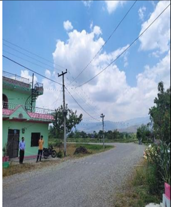
Figure 4: Photos during Structure Verification - Duimat Chowk-Tali Section
