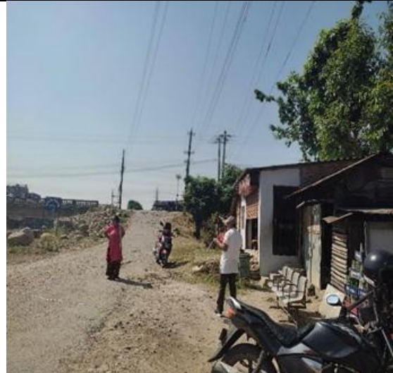
Figure 4: Ending Point, Affected Structures of Tej Bahadur Pun (Right Side) Chainage 9+440
