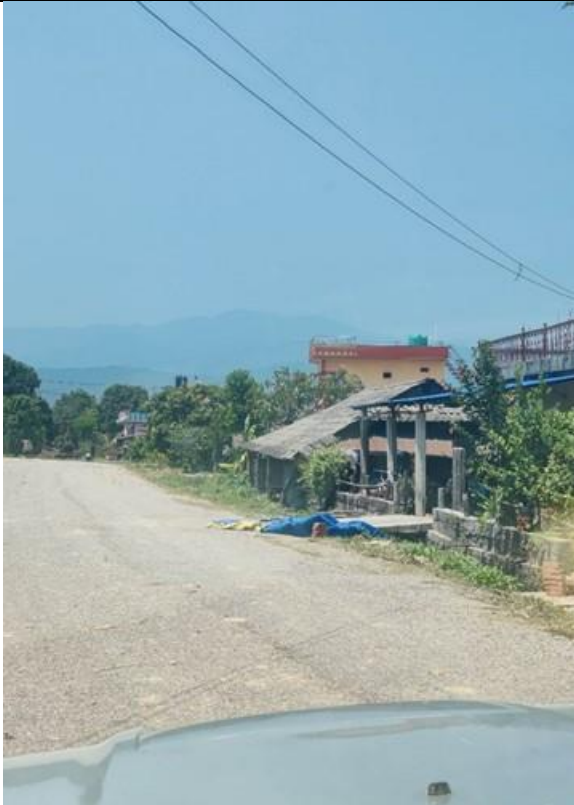
Figure 3: Affected shed of the alignment
